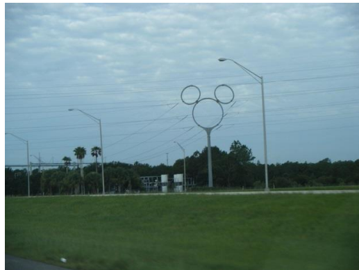
Transmission Tower near Celebration, Florida
